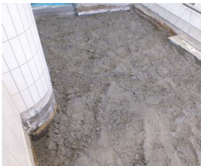
Installation of a composite surface in a industrial kitchen
