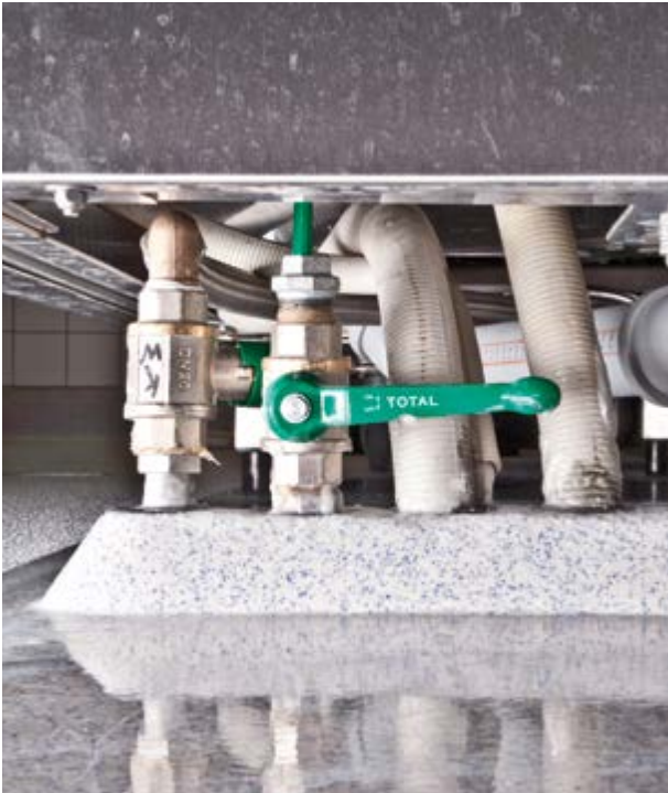
Interrupting element with triangular base/plinth
