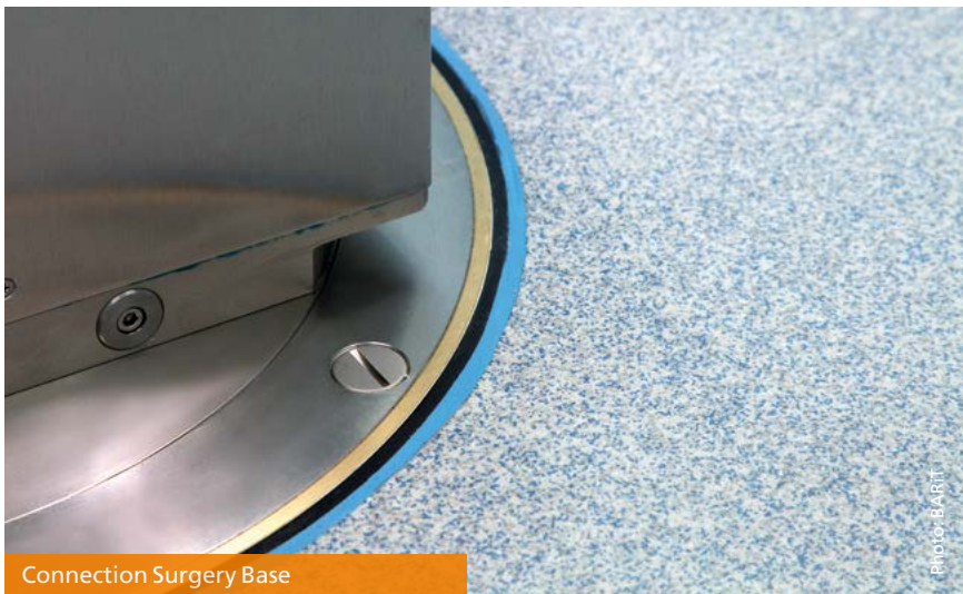
BARiT ATEX-TERRAZZO, electrically conductive | Clean Room Floor | Kinderklinik Aschau
