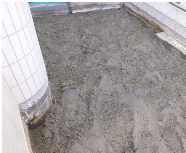
Installation of a composite surface in a commercial kitchen
