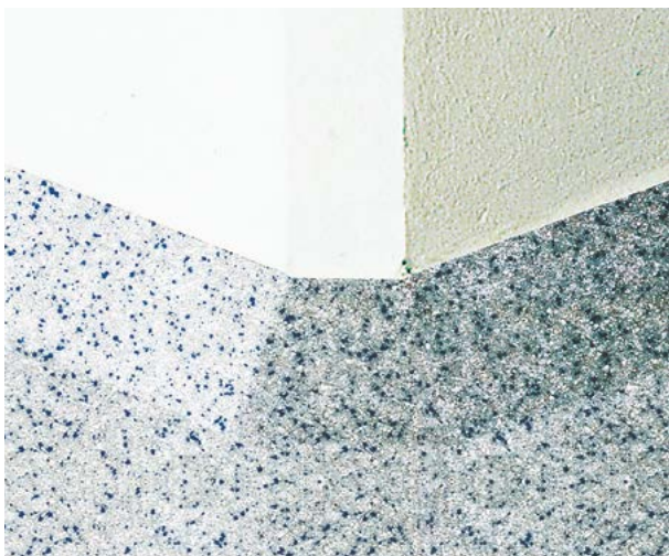
Triangular base/plinth is accurately modeled by hand
