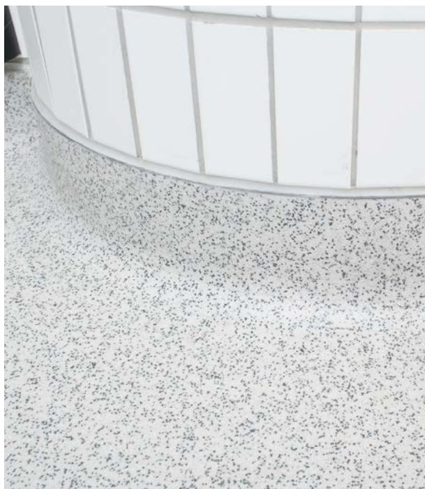
Channels for the composite are modeled into a smooth surface on the pillars.
