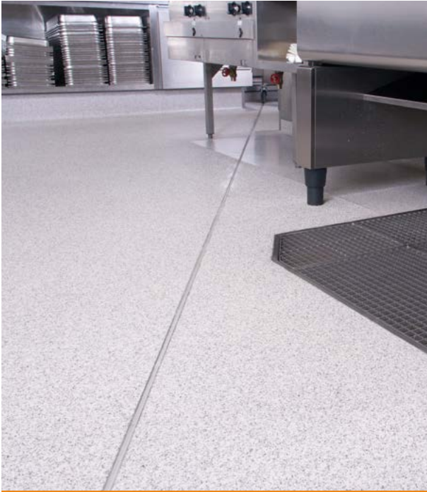
Expansion joints are installed in resin concrete.
