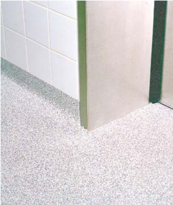
Prefabrication of a coving for a surgical doorframe
