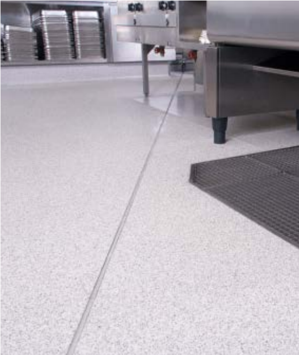
Expansion joints are installed in epoxy cement concrete
